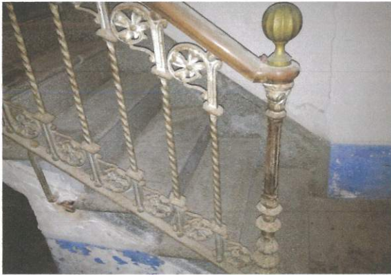
Barana escala interior
